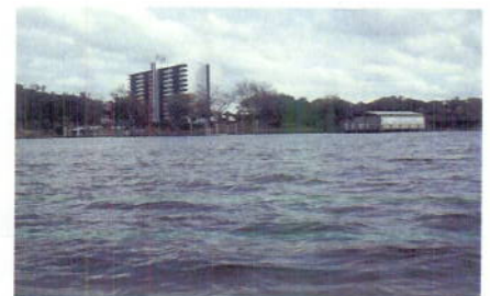
Riverton Tower from St. Johns River
